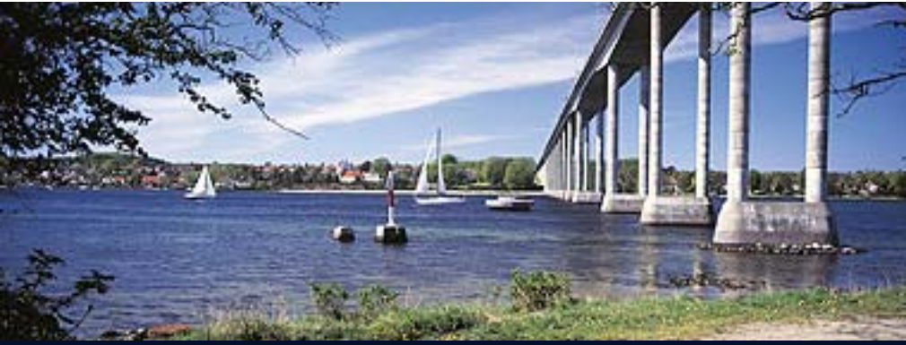
Svendborgsund Bridge 1966. Part of the fixed road link between Denmark's third-largest island, Funen, and the smaller islands Tåsinge, Sjø and Langeland, the concrete box girder bridge is 1,220 metre long with 33 metre clearance. Photo: Preben Eider.
