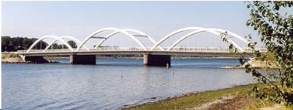
Munkholm Bridge 1952. The purpose of many small road bridges across bays is to reduce distances. The arched bridge is 114 metres long with 3 metre clearance. Photo: Unknown.
