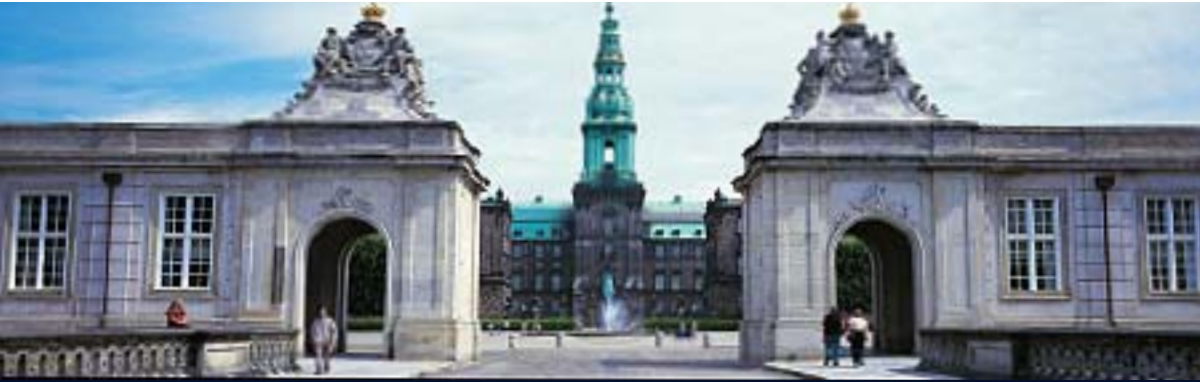
View of the Danish Parliament building, Christiansborg Palace, which is situated on the small island of Slotsholmen located in central Copenhagen.
